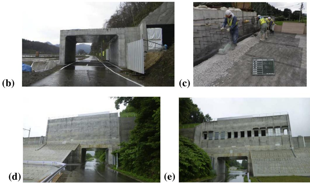
Fig. 21. RC box culvert at site B1 in front of the entrance of Shin-Moheji tunnel: (a) construction sequences (1) – (10) (stages (2) & (6) are not indicated); and views (b) after stage (6); (c) during stage (7); and (d and e) completed.
