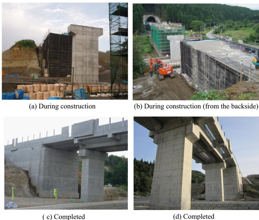
Fig. 11. GRS Bridge Abutment at Mantaro (A21 in Fig. 2).
