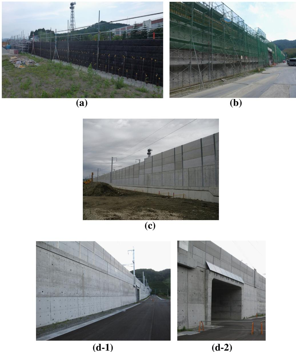
**Fig. 4.** GRS RW with FHR facing before stage 6; (a) at the western side of the GRS Integral Bridge at Kikonai; and (b) at both sides of box culvert B2; and (c and d) completed GRS RWs.
