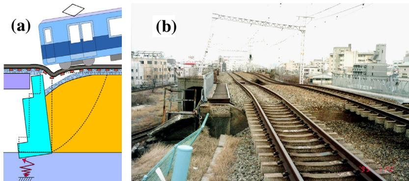
Fig. 8. (a) Illustration of a large bump behind the conventional type abutment; and (b) a typical case near Shin-Nagata Station of JR Kobe Line during the 1995 Kobe earthquake.
